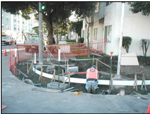
Installing Code Compliant Curb Ramps
